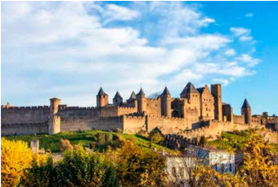
Figure 1: The city of Carcassonne in France is a concentric castle, featuring multiple layers of curtains walls.
